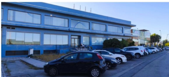
Main façade of the Dávila Building.
